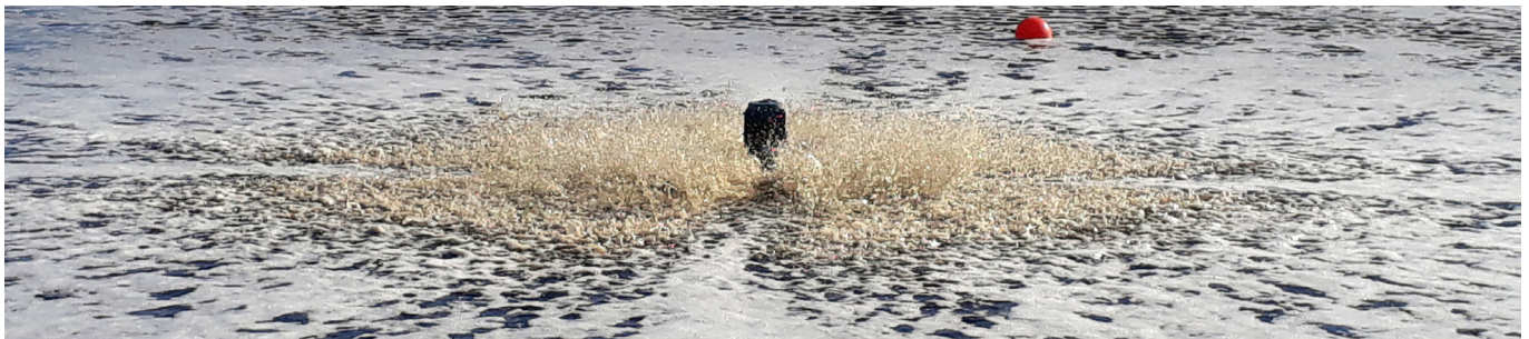
Water aeration in an equalization basin.
